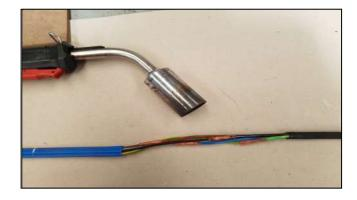
Clean and degrease the previously abraded outer sheaths.
