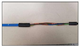
Position outer sealing sleeve centrally over the joint area.
